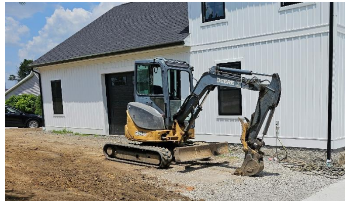
Figure 1 – Southwestern wall and driveway area of 329 Haymond St; note the door behind the small excavator
