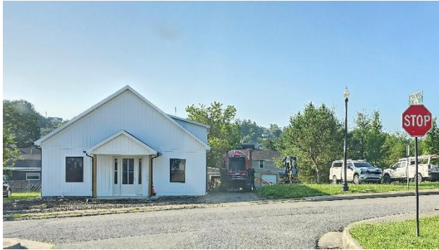
Figure 2 – Looking at the front door and driveway of 329 Haymond St
