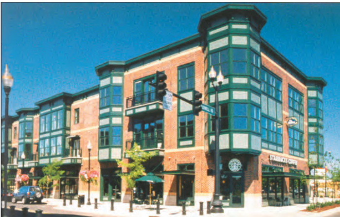
Buildings with consistent character and quality are important to defining districts and establishing a unique aesthetic quality.
