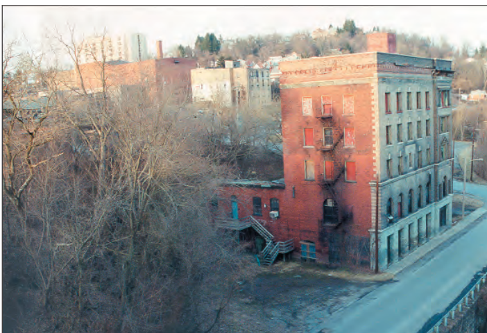
Many historic buildings in the RA have fallen into disrepair and are vacant or underutilized like the former Elks Lodge at the intersection of Madison Street and Cleveland Avenue.
